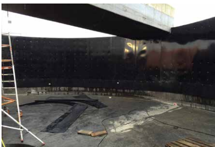
PE-HD vlakke renovatiebeplating
